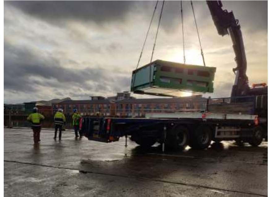
Second weight basket being unloaded at site followed by plinth/tower interface 16 th December
