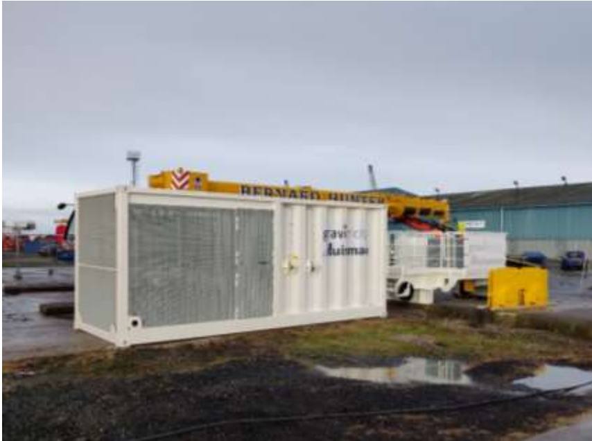
Top frame, winch container and lower sheave blocks at demonstrator site 14 th December
